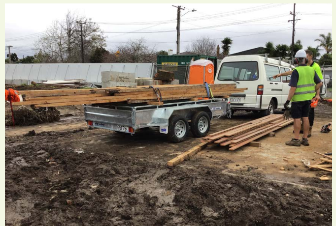
Timber extracted for reuse from the Martin Leone houses.
